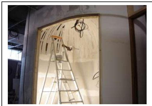
Figure 5: Construction. Outside view
