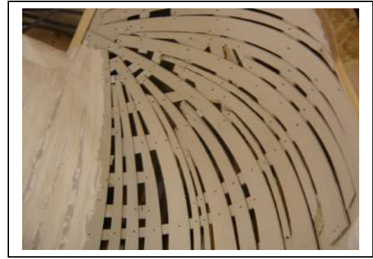
Figure 6: Construction of the domed ceiling
