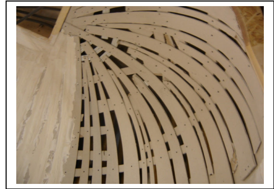
Figure 6: Construction of the domed ceiling
